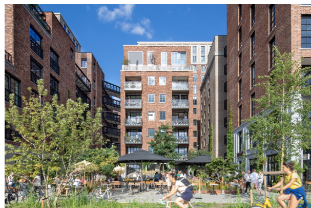
Coolhaven in Rotterdam, door Little C.
