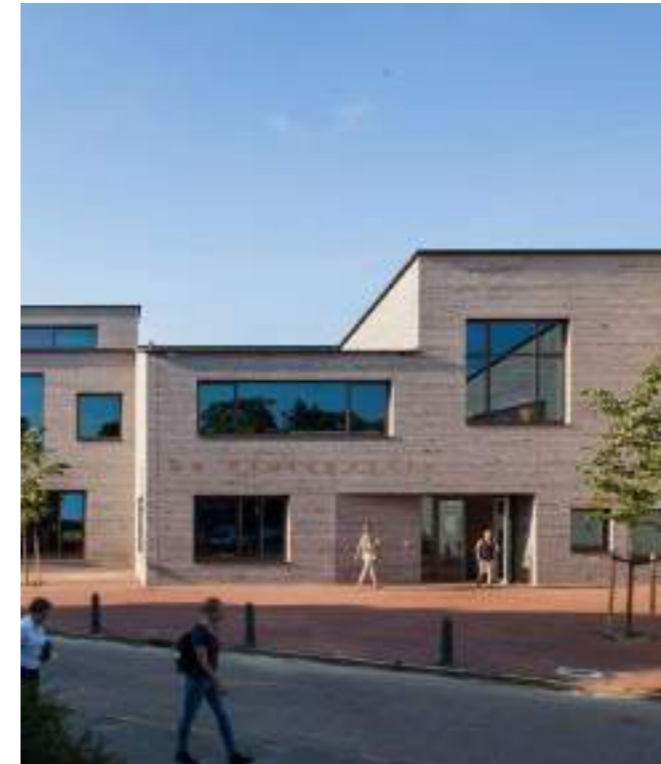
Combinatie van baksteenstructuren Mellor Primary School, Leicester
